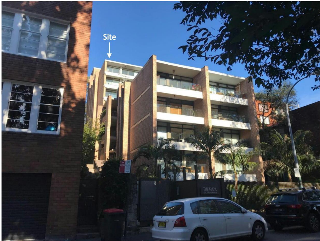
Figure 7: View of subject site from Billyard Avenue
