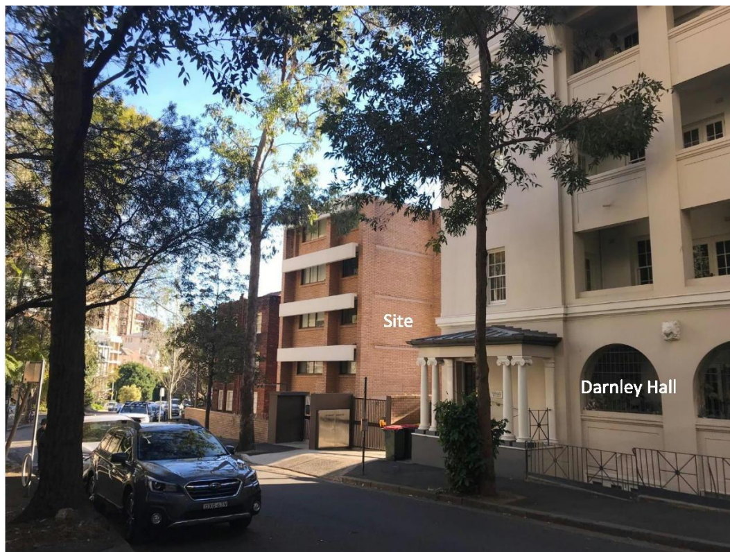
Figure 2: Site viewed from Onslow Avenue looking north
